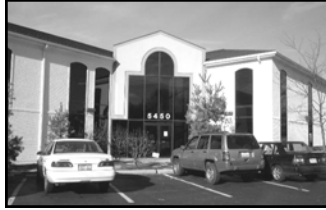
Rahn Fountain Plaza, Kettering 200sf - 2,279sf Office Space For Lease
