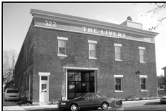
The Livery (322 S. Patterson), Dayton 450-5,376sf Office Space For Lease, Building For Sale
